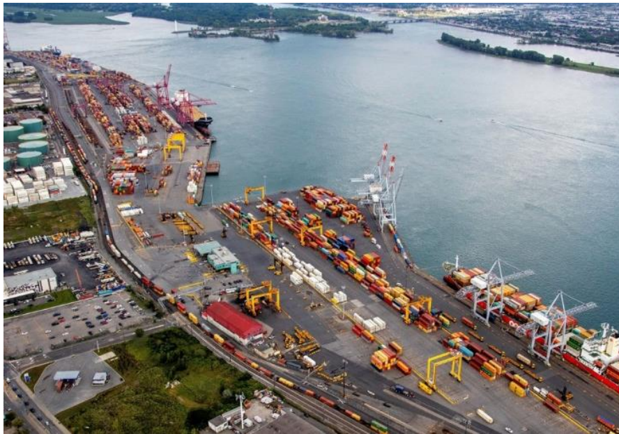
Figure 30 Port of Montreal
