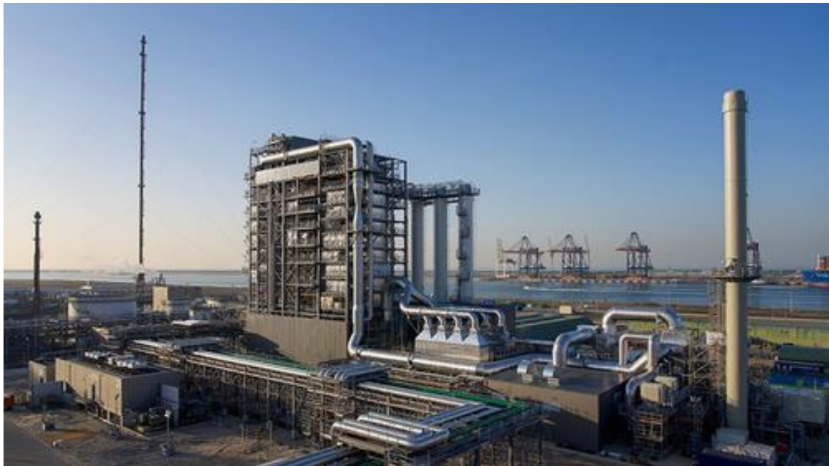
Figure 15 Bio plant and incinerator converting water-based waste to energy in Rotterdam
