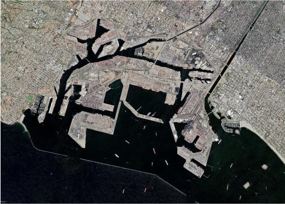
Figure 22 Port of Long Beach Aerial View
