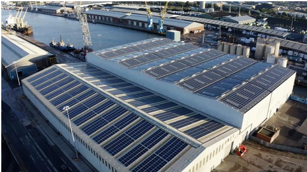
Figure 32 Solar panels at Southampton Port
