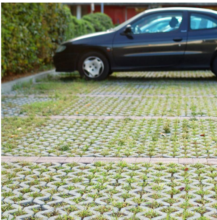
Picture 29. An example of a parking lot with a higher permeability of the material (photo: https://www.respectourwaters.org/pervious-pavement )
